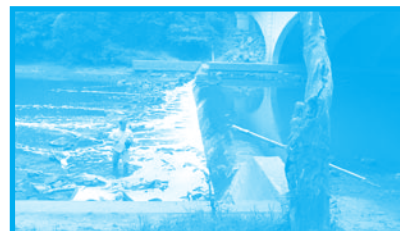
Highland Park Dam Before (top): The low-head dam caused a dangerous flow pattern on the downstream side that blocked fish passage and could trap waders.
