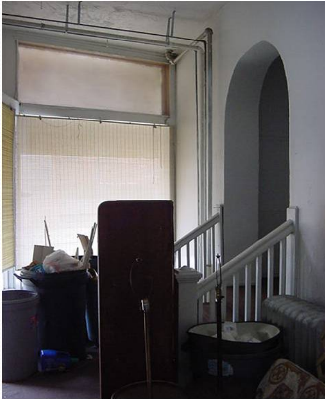
Lobby Before Renovations
